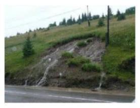
The development of roads and structures changes the movement of water, causing erosion.
